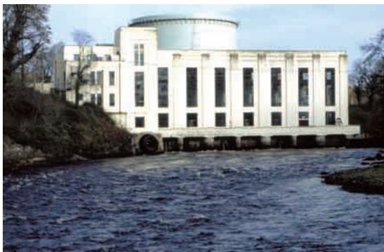
Tongland Power Station
